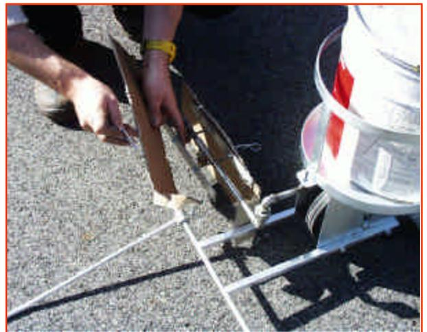
**Fig 5:** Fixing spray protection cardbox
